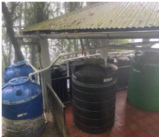
Rain water harvesting system from roof of the college building and water Distribution system
