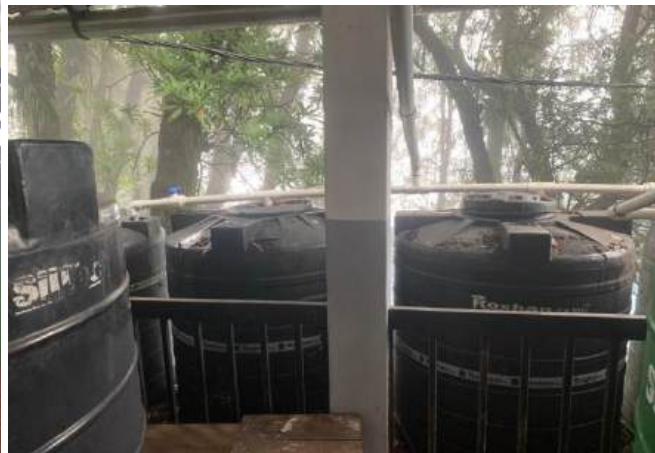
Rain water harvesting system from roof of the college building and water Distribution system
